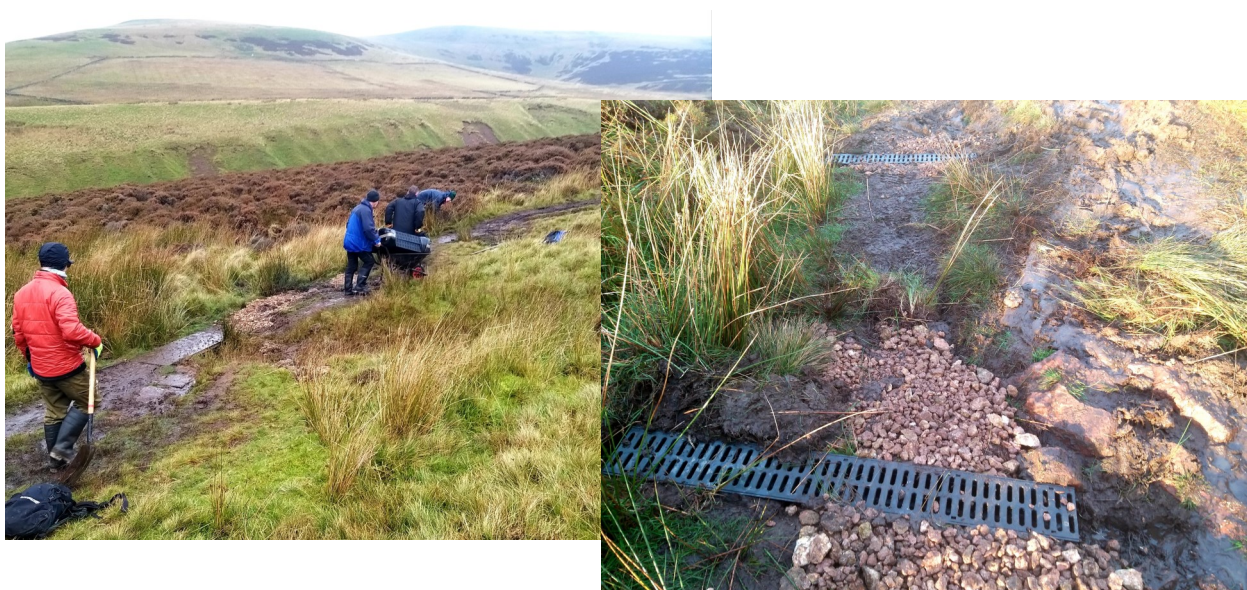
Drainage works on the Kirkburn Path: Photos Donald Sandeman
