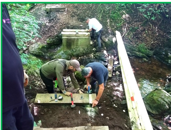
Bridge repairs at Bonaly
