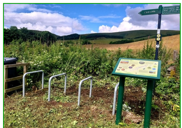
Bike rack installation at Nine Mile Burn
