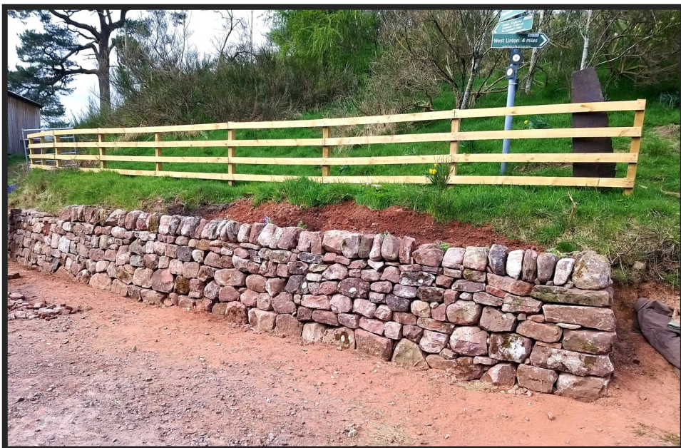
Photographs of Friends volunteers building a drystone dyke at Garvald
