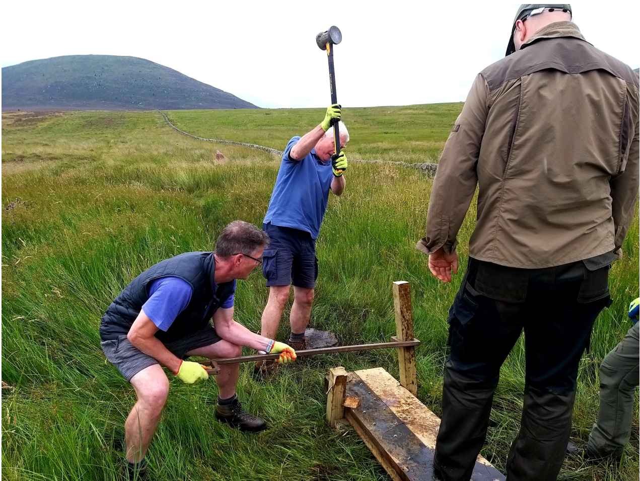
Get a grip! A work Party installs a bog bridge on the Thieves Road
