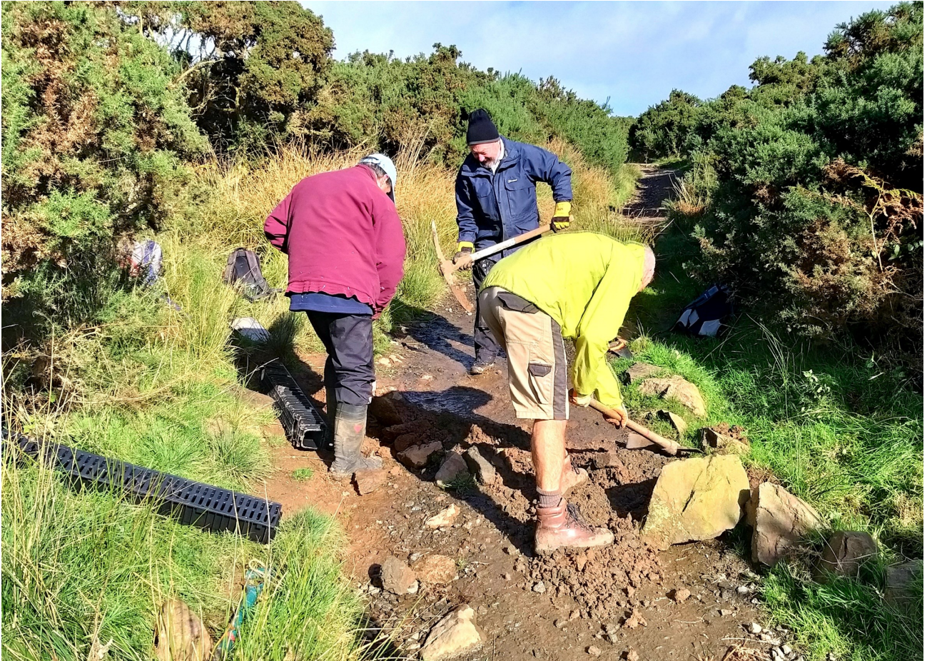
Draining work on Buckie Brae
